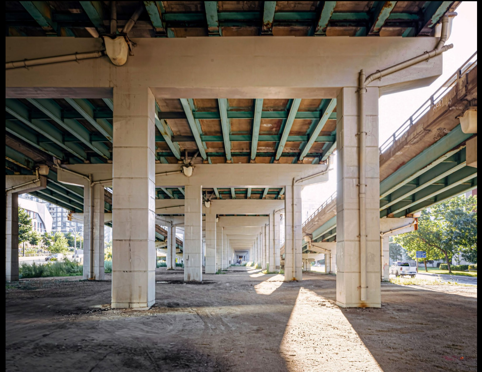
Future site, The Bentway Islands
